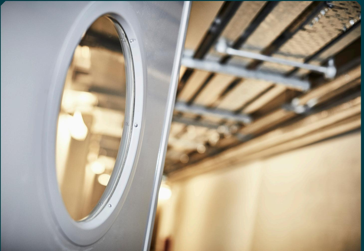
The Defender Fireshield doorset has been successfully tested at Exova Warrington Fire to BS EN 1634-1:2008 in January 2014, Test No: WF336507. Available with many ironmongery combinations and glazed options.
